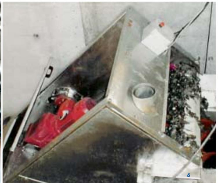
It is for this reason, that the amount of waste water required is pumped from the main channel, cleaned in a two step process (mechanically and by sedimentation) and finally is passing through the shell and tube heat exchangers of the two heat pump units.
